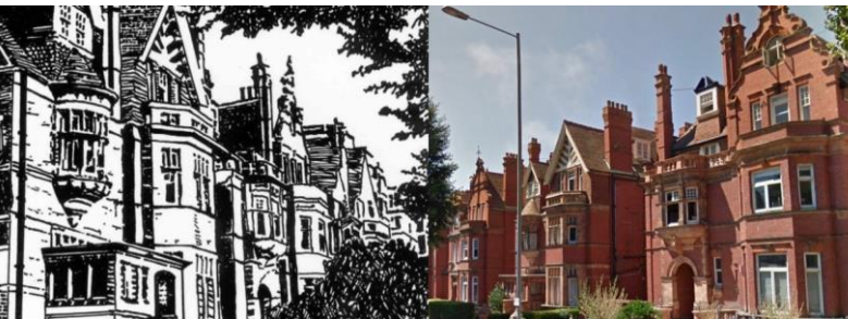
Figure 14 - The Drive Conservation Area
