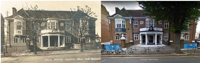
Figure 15 - Ralli Memorial Hall, walls and railings grade II; the design is in the 'Wrenaissance' style, with red brick walls laid in English bond, a hipped clay tile roof with upswept eaves and a strongly moulded wooden dentil cornice.
