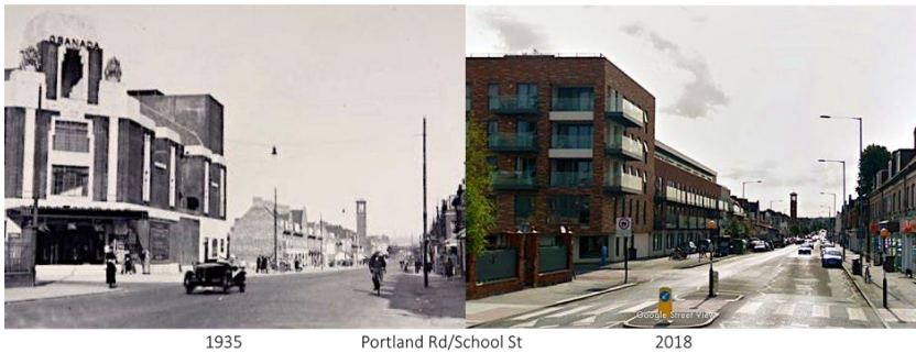
1935 Portland Rd/School St 2018
